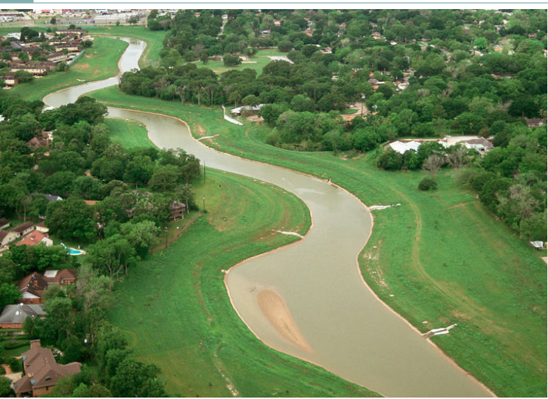
Restoration of Sims Bayou in Houston, Texas consisted of earthen channels and tree plantings to reduce flood risks. Photo: SWA Group
