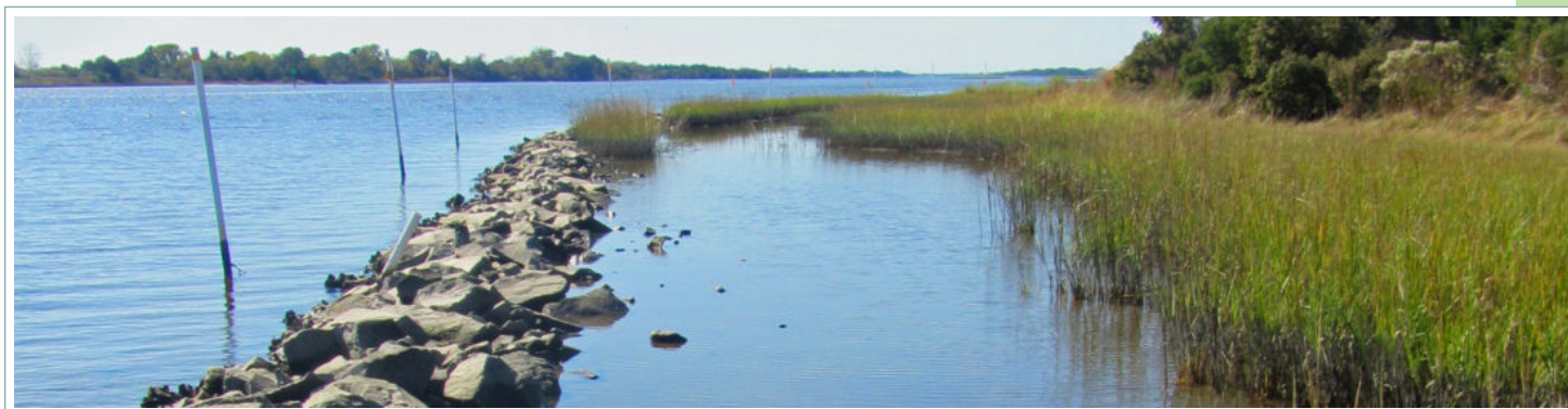
Living shorelines with rock sills can enhance salt marsh resilience to erosion and storms. Photo: Carter Smith
